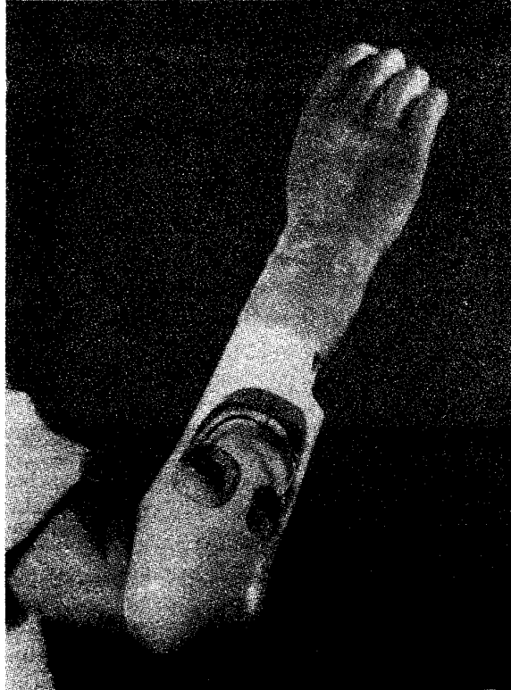
Fig. 1. Sauerbruch - cineplastic controlling an electric hand prosthesis
